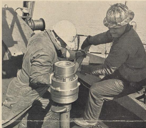
Crew members of drilling ship Simcoe tighten head onto length of pipe as production well is sunk towards gas reservoir a thousand feet down in sandstone.
