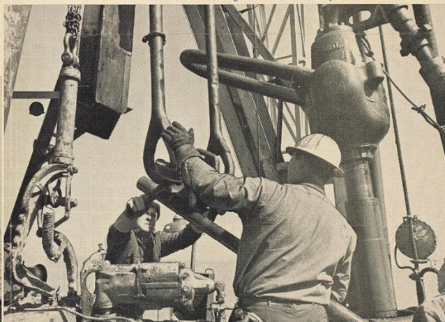
Another section of production pipe is brought to drilling tower from the stock piled on the deck of the Simcoe . In 1961 the drilling ship lost her 90-foot tower and superstructure in a gale of wind.
