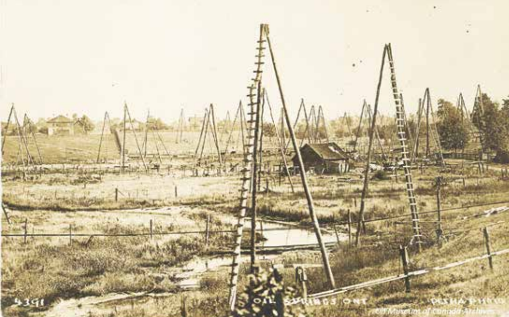
Figure 3: Tripods set up over wells drilled along Black Creek in the Oil Springs Oil Pool. The tripods are used to lift and lower drilling tools in and out of the well (Photo courtesy of the Oil Museum of Canada Archives).
