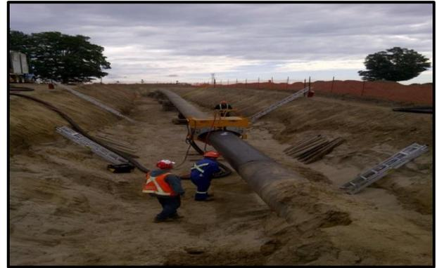
Figure 2: Pipe Viper machine stripping old pipe leaving behind a smooth pipe with no coating on the surface
